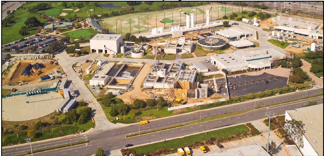
Figure 8-1 West Basin’s Water Recycling Treatment Plant
