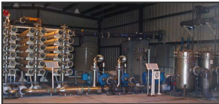
Brewer Desalter RO treatment on-site
