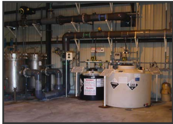
Chemical addition tanks located inside the RO building
